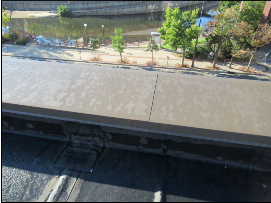
9. Short parapet wall cap flashing.
