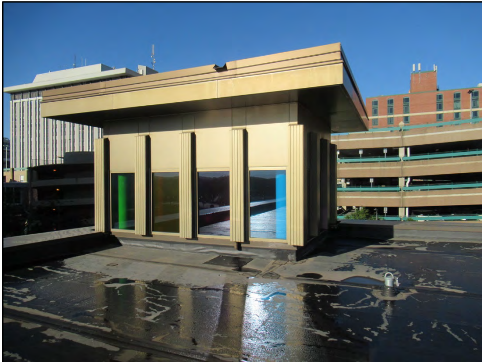
10. Lantern as the southwest corner of the roof.
