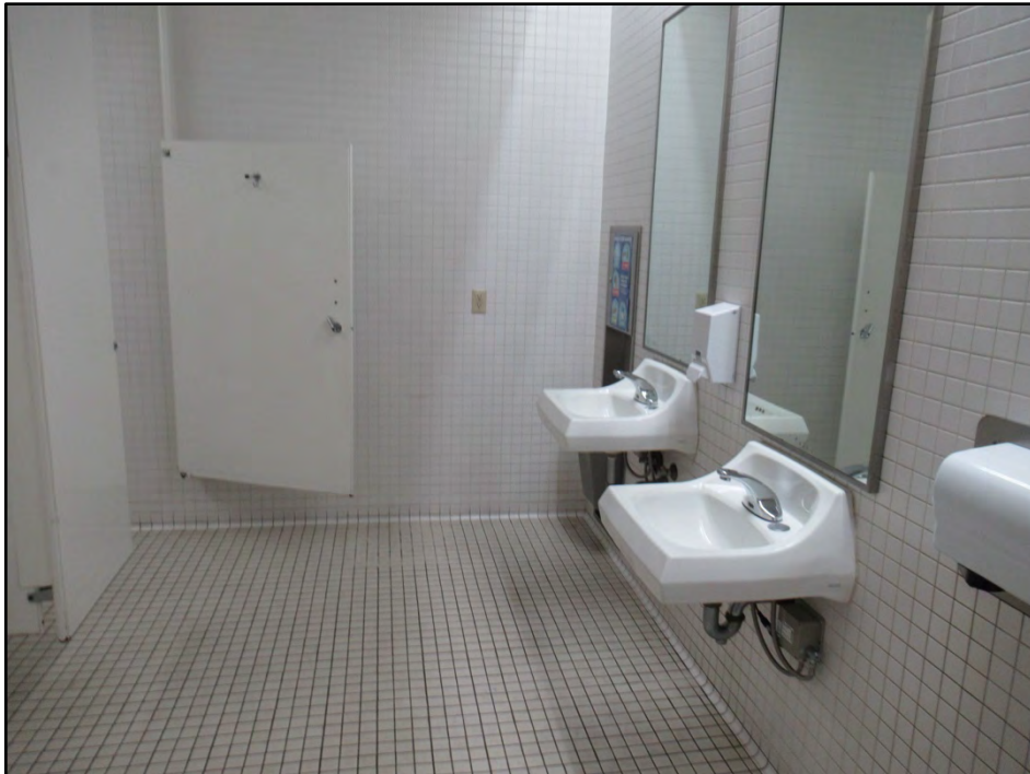
28. Restroom interior finishes.
