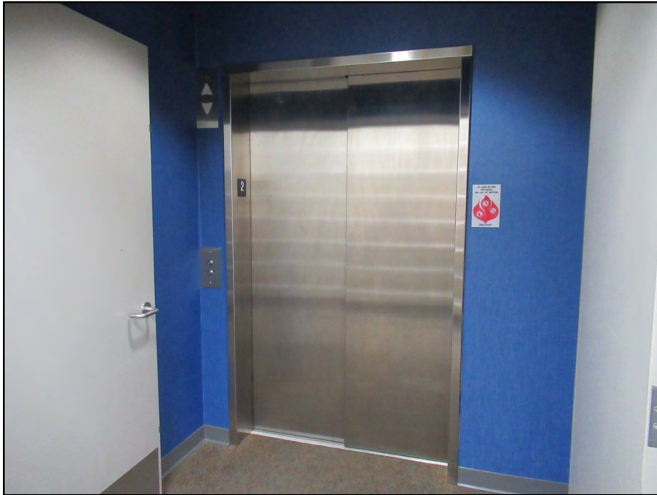
37. Service / passenger elevator lobby 2 nd floor.
