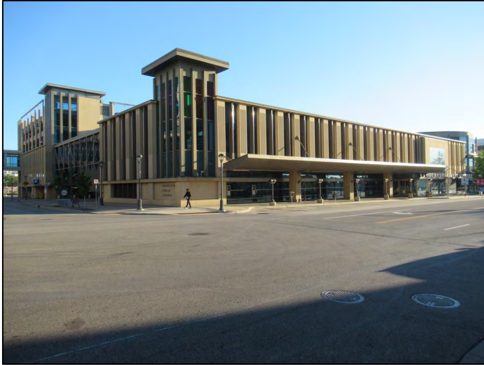
1. South and west elevations as seen from 2 nd Street.
