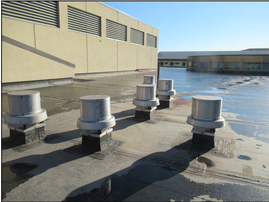
7. Overview of the roof looking east.
