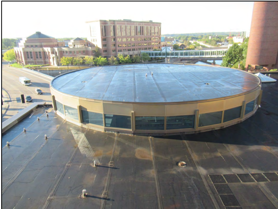
8. Overview of the roof looking south.
