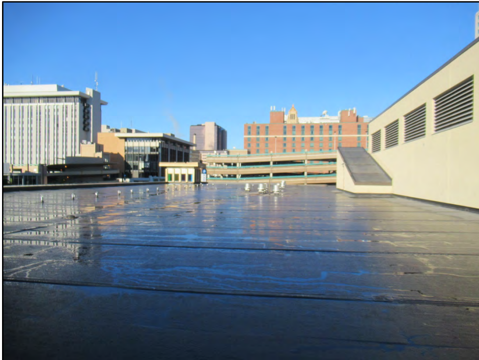
6. Overview of the roof looking west.
